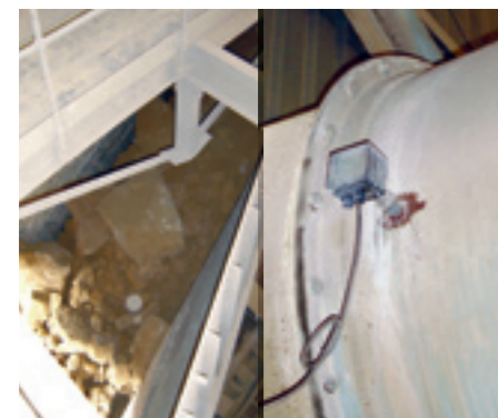
Crusher plant filter protected by an advanced Electrodynamic unit
