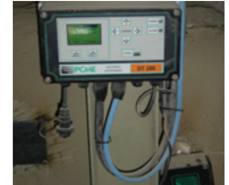
Product loss prevented by silo monitoring
