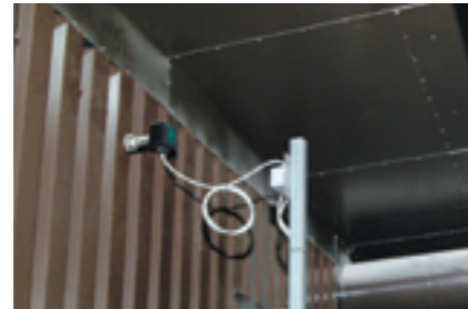
Filter chamber performance continuously monitored via a networked Electrodynamic system
