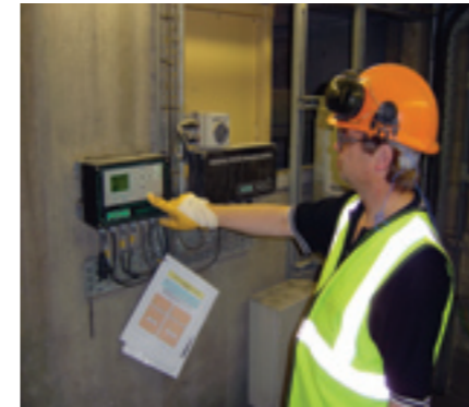
Filter condition assessed remotely
